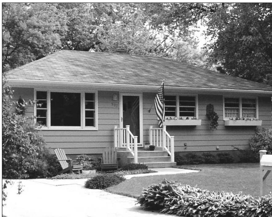
This ranch-style home has 224 ft 2 of original wood, single-pane, mostly double hung windows.
