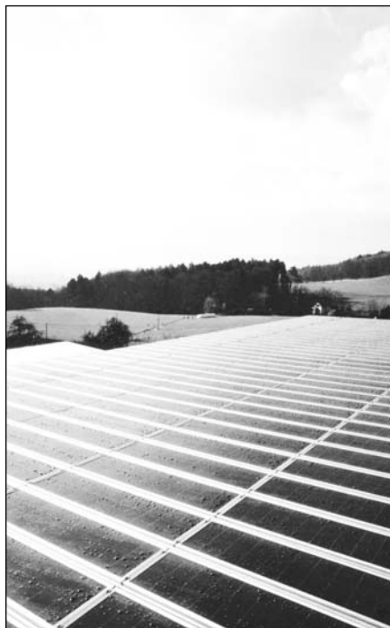
(left) The entire roof of Sunny Woods is covered by PV panels, yet the integrity of the roof is not compromised by penetrations into its aluminum surface. (right) Only the garage and basement of Sunny Woods are made of concrete. Red cedar from Oregon was chosen for the façade.
