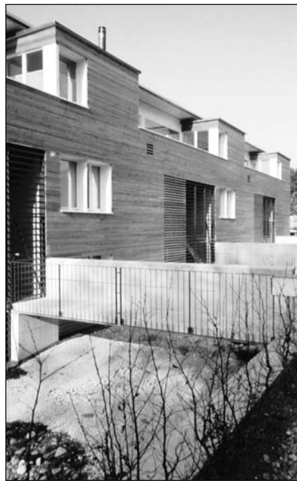
(left) The entire roof of Sunny Woods is covered by PV panels, yet the integrity of the roof is not compromised by penetrations into its aluminum surface. (right) Only the garage and basement of Sunny Woods are made of concrete. Red cedar from Oregon was chosen for the façade.
